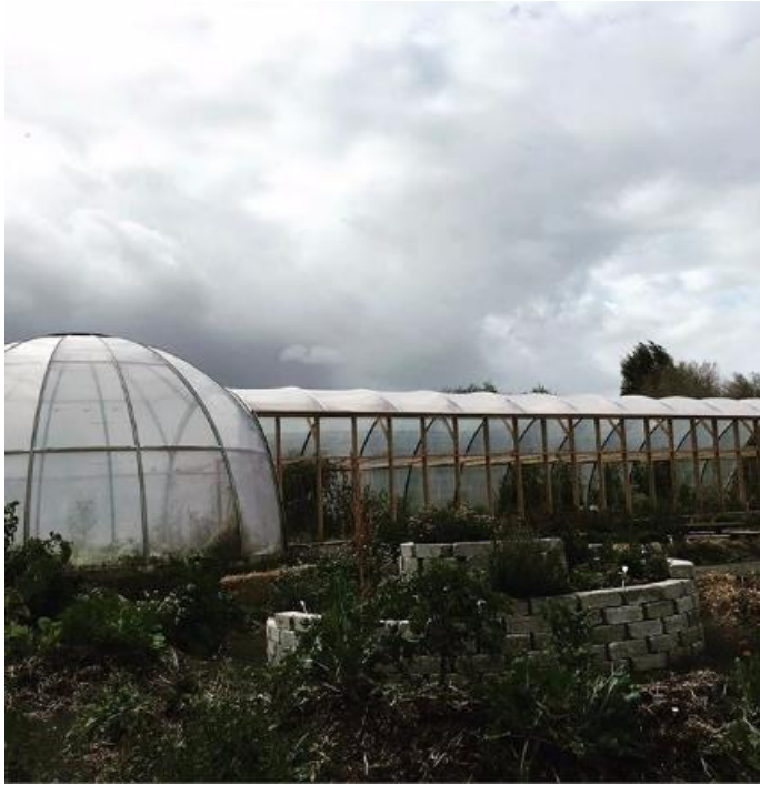
Figure 3 The greenhouse by the restaurant
