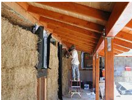
Figure 1 Building a straw bale house
